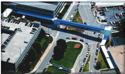
Decatur VA Pedestrian Bridge - Decatur, GA
