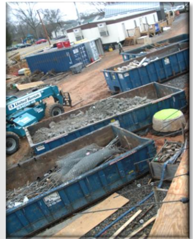
Over 1532 tons of waste diverted On Hotel Indigo - Athens, GA
