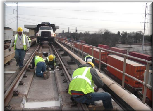
MARTA Grout Pockets - Heavy Construction
