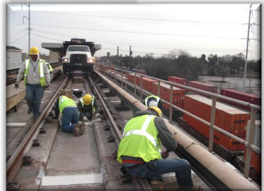
MARTA Grout Pockets - Heavy Construction
