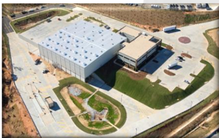
DeKalb County Transfer Station - Atlanta, GA
