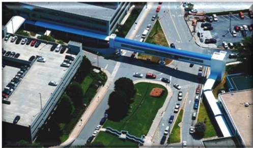
Decatur VA Pedestrian Bridge - Decatur, GA
