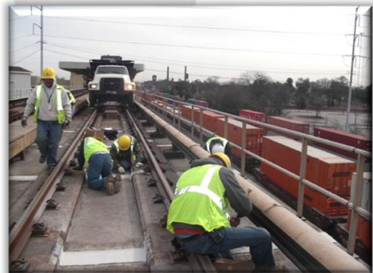
MARTA Grout Pockets - Heavy Construction
