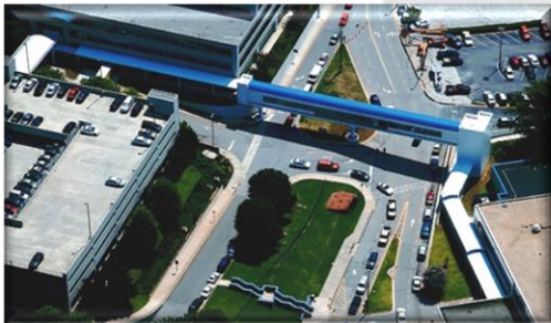
Decatur VA Pedestrian Bridge - Decatur, GA
