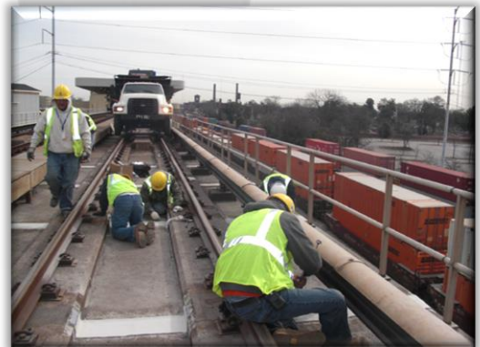
MARTA Grout Pockets - Heavy Construction
